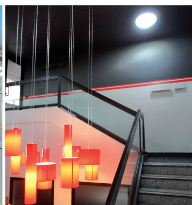
Office building with light pipes, Lightway, Czech Republic
