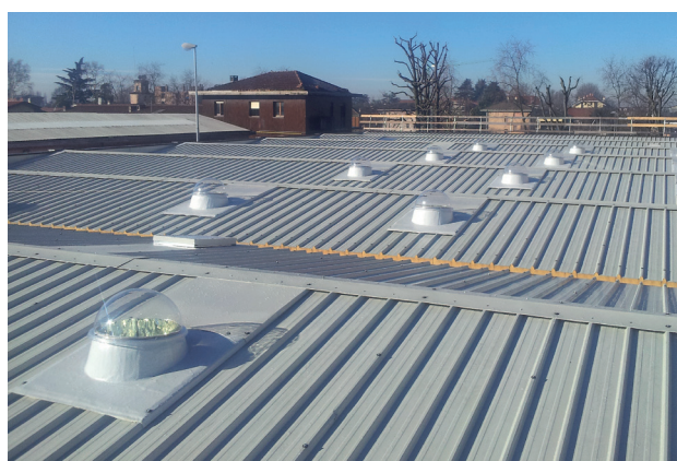
Roof at Gimec, Baggilux, Italy
