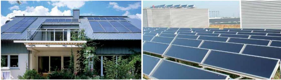
The TiNOX absorbers are energy traps. They collect almost all available solar radiation and convert it into heat. Unlike black chrome or black-coated absorbers, almost none of this energy is lost again as heat radiation. The energy is directly transferred into the heating-support and water heating systems by the TiNOX absorbers. **The energy trap**
